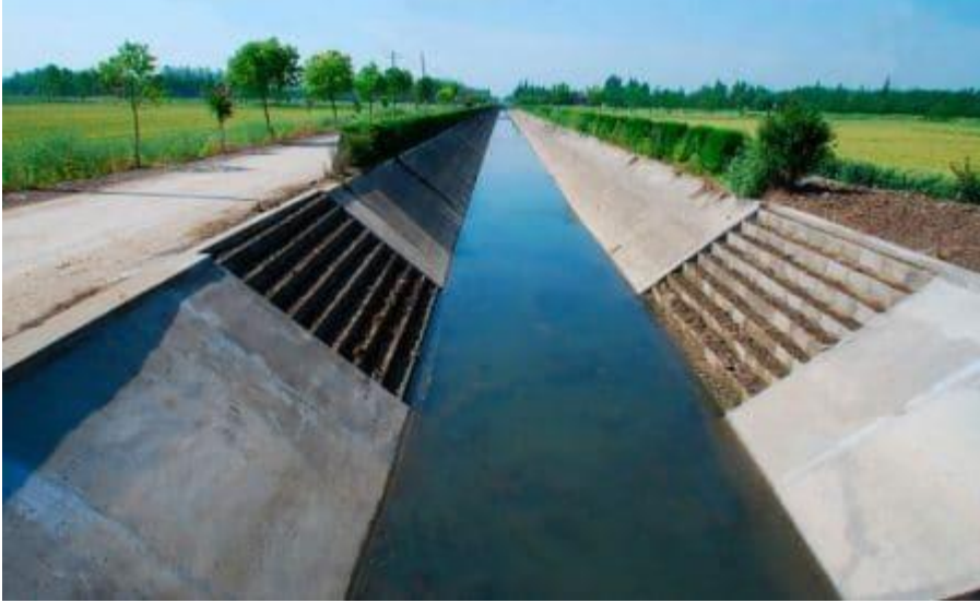
Fig 9: Rigid Surface Canal or Lined Canal
