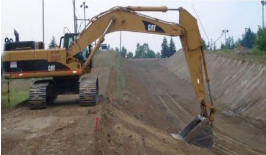
Fig 2: Compacted Earth Lining
