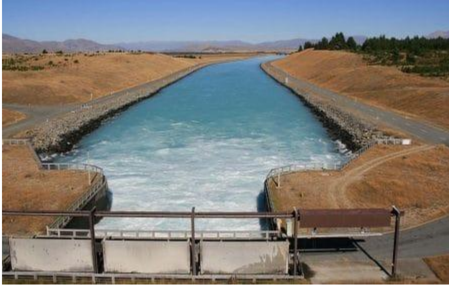
Fig 3: Power Canal of Lake Tekapo, Newzeland
